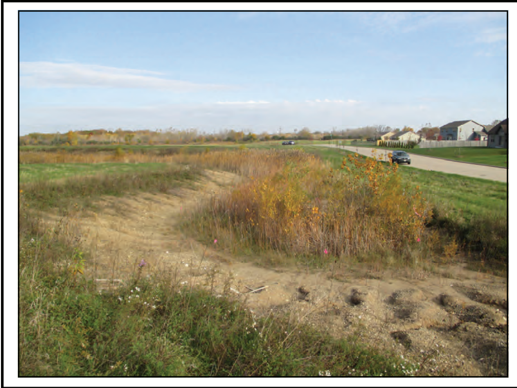
Photograph 3 (10/21/14): North facing view of the south end of W-3. W-3 is a man-made drainage feature that conveys water westerly into the stormwater pond.
